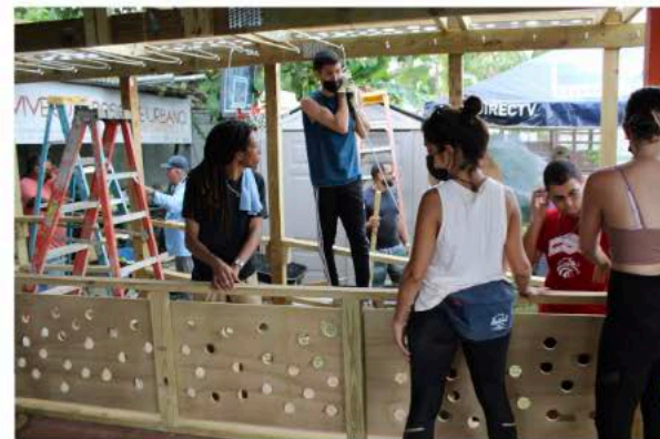
Co-design/build Pergola in situ
