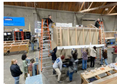
CAPLA students building a tiny home - Sound Foundations NW
