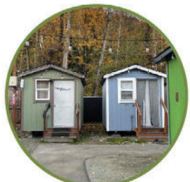
Sound Foundations NW Shelter
