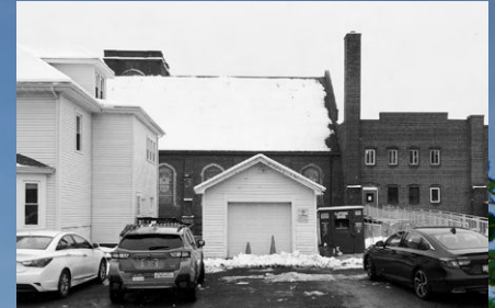
EXISTING CHURCH + PARSONAGE
