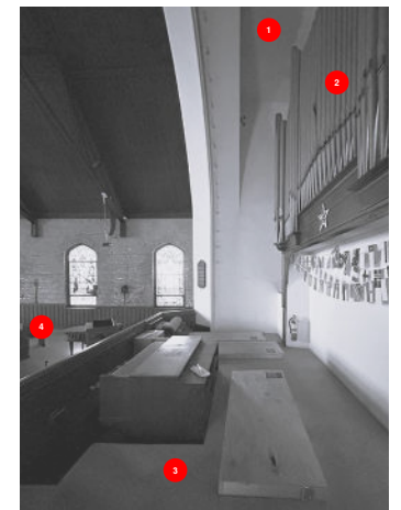
EXISTING CHANCEL ARCH
