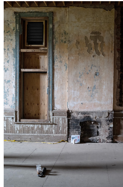
OLD YMCA: stabilized interior
