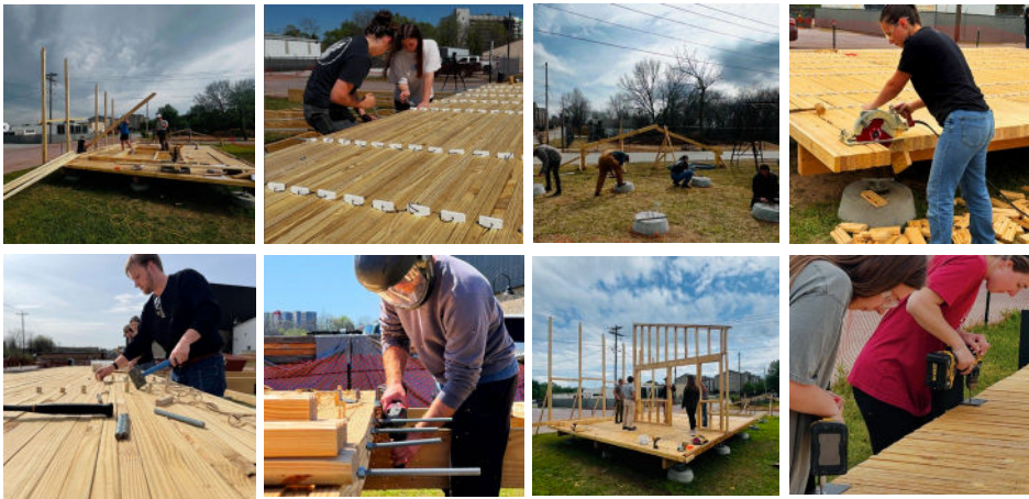
LEFT: Images of UDBS AR HOME CoLAB students engaged in the construction of the public demonstration of the UNTITLED HOME v01 prototype. Activities shown include tilting up columns, installation of custom steel column connectors, and the continuous tightening of threaded tension elements through strategically placed port holes in the WLT deck assembly. The work provided hands-on job-skill training in precision timber fabrication, post-tensioning systems, finish detailing, and tool safety, offering students real-world experience in both innovative and conventional construction practices. RIGHT: Examples of student work: drawings to guide the construction of the WLT deck assembly, framed walls, and WLT bent members.
