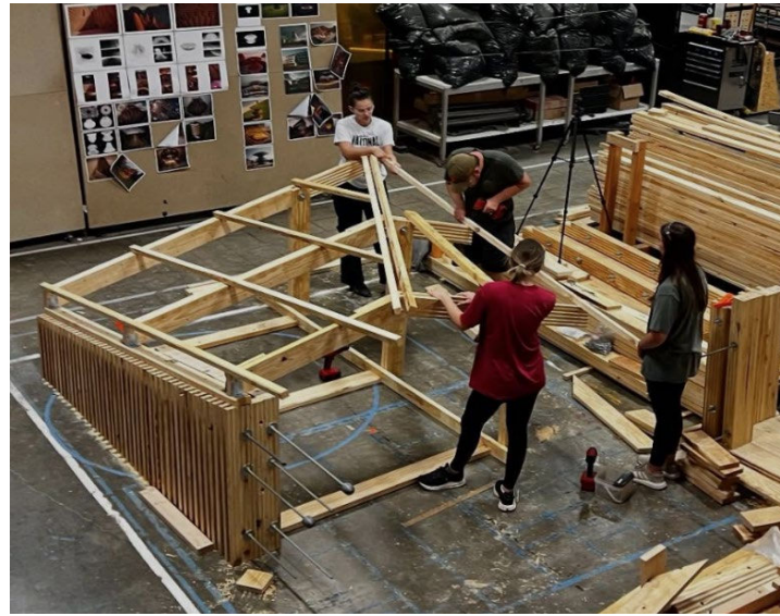
3D digital model views and construction images of a large-scale mockup of the UNTITLED Home prototype under assembly by students. The mockup includes key structural systems of the prototype, including the Wave-Layered Timber (WLT) cavity wall, laminated WLT columns, structural bents, and portions of the roof assembly constructed at full scale.
