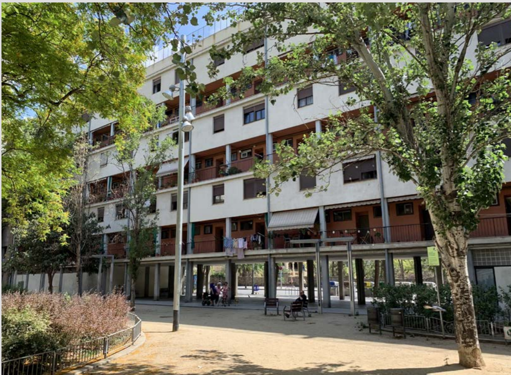
Sert and GATCPAC, Casa Bloc housing for textile workers, Barcelona, 1932-35
