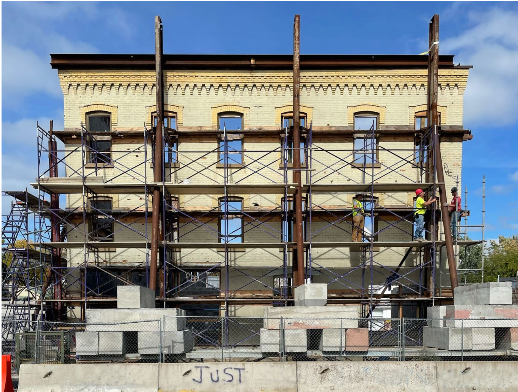
Ironworks Building Facade After Disassembly
