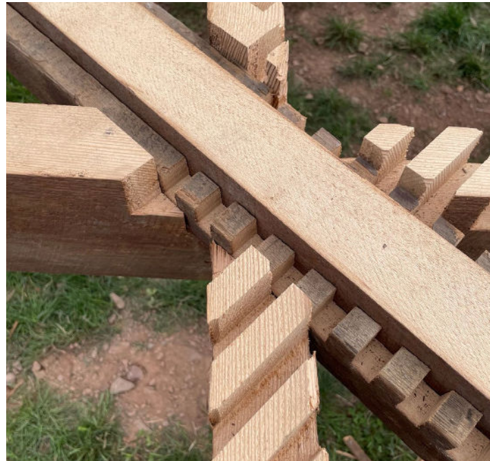
CNC Tolerance + Joinery Details
