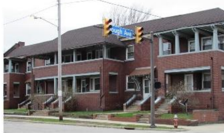
MULTI-FAMILY RESIDENTIAL REHABILITATION HOUGH AREA DEVELOPMENT CORPORATION CLEVELAND, OHIO 1979
