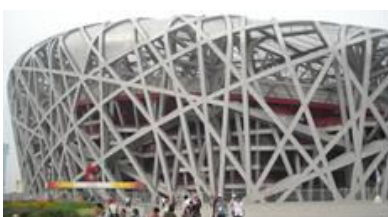
OLYMPIC STADIUM (BIRD'S NEST), BEIJING
