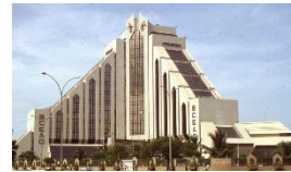
Bank of ECOWAS, Dakar Goudiaby,Architect
