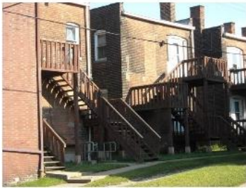
MULTI-FAMILY RESIDENTIAL REHABILITATION HOUGH AREA DEVELOPMENT CORPORATION CLEVELAND, OHIO 1979
