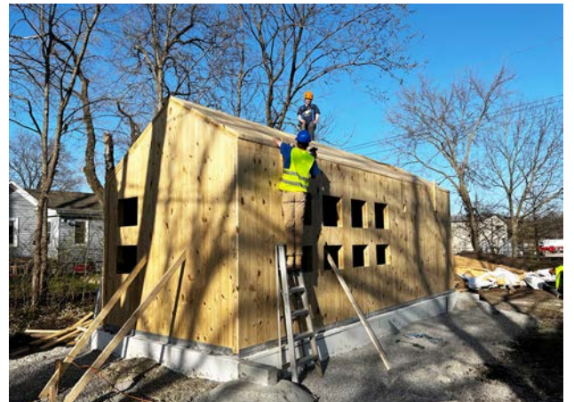
cross laminated timber shell in place with minor adjustments
