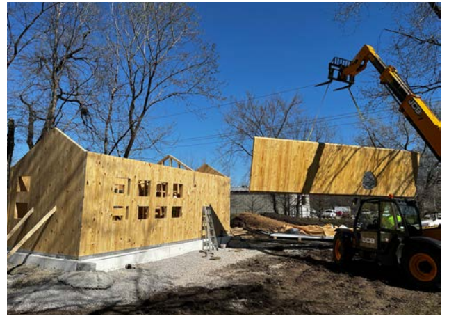
a cross laminated timber roof panel is lifted into place
