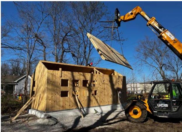
the final cross laminated timber roof panel is being installed
