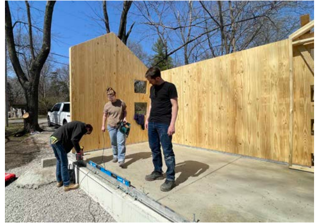
cross laminated timber panels are install, one-by-one
