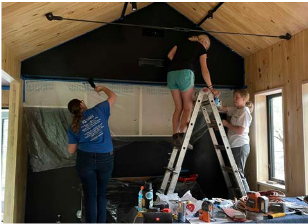
painting, trim installation, countertops, MEP finishing
