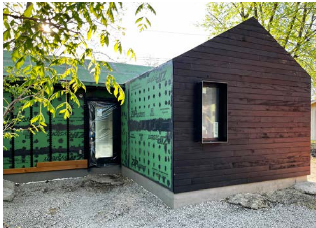
rain screen installation continuing
