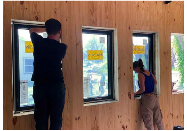
windows and doors are installed
