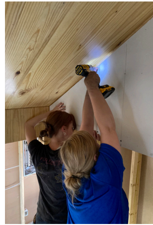
drywall is installed, mudded, and CLT walls clear coated
