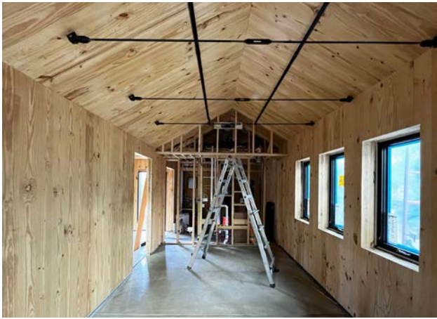
framing, windows, doors, and MEP rough-in complete
