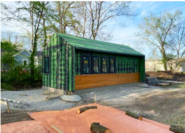
rainscreen clip system installed and rain screen beginning
