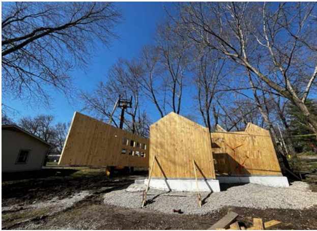
the final cross laminated timber wall panel is being installed
