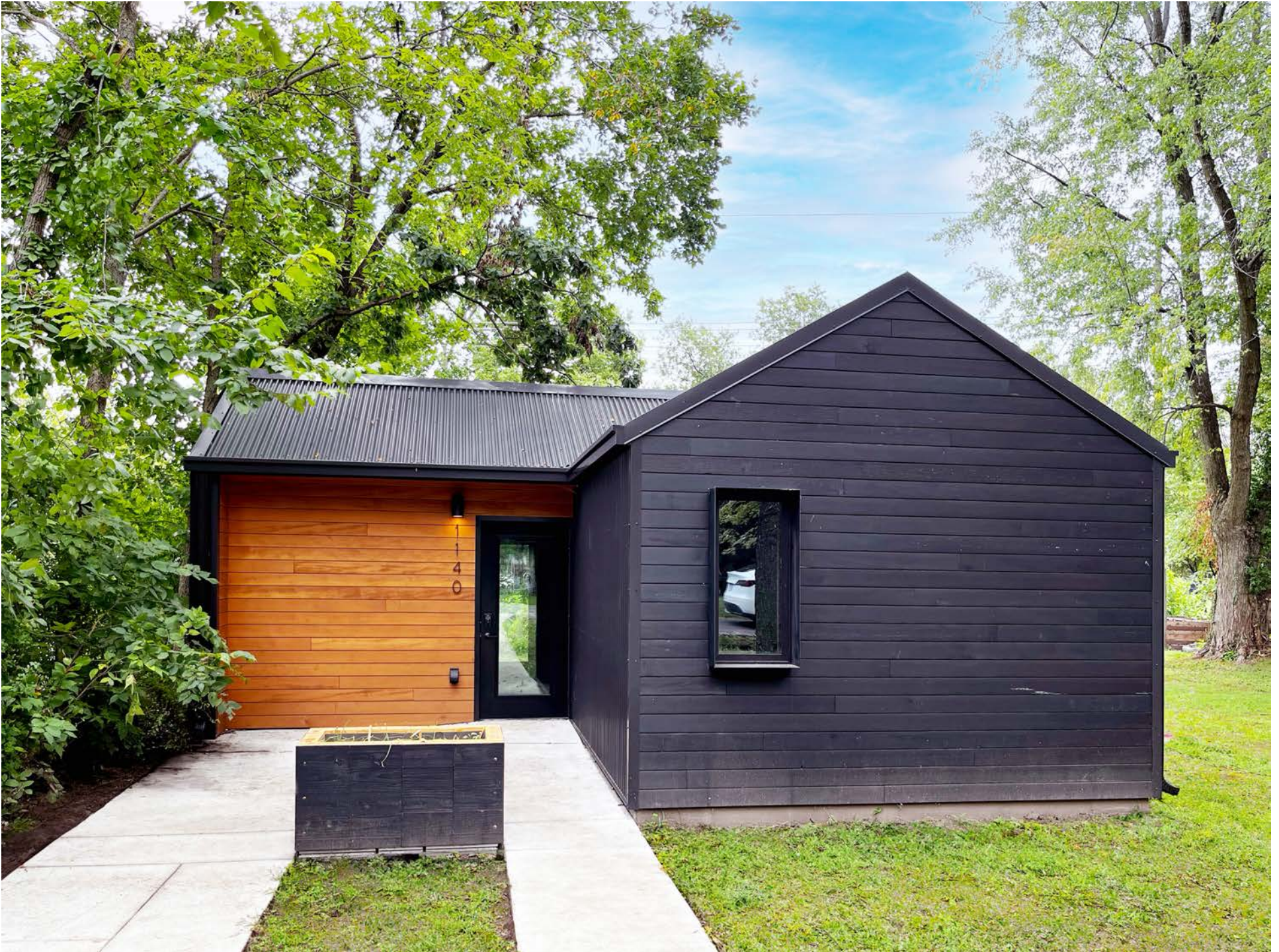
Exterior view of the street-facing west facade, with a CLT planter defining a front entry space and a protruding window offering views to the street while preserving privacy
