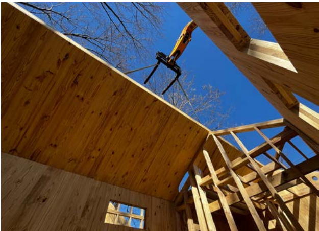
the cross laminated timber roof and wall panels are fastened
