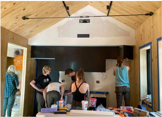
drywall wall is finished and sanded, cabinetry installed
