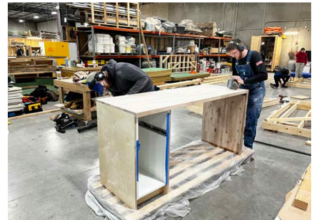
prefabrication of custom kitchen island/dinning bar
