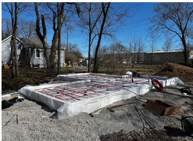
installed foundation insulation and radiant tubing
