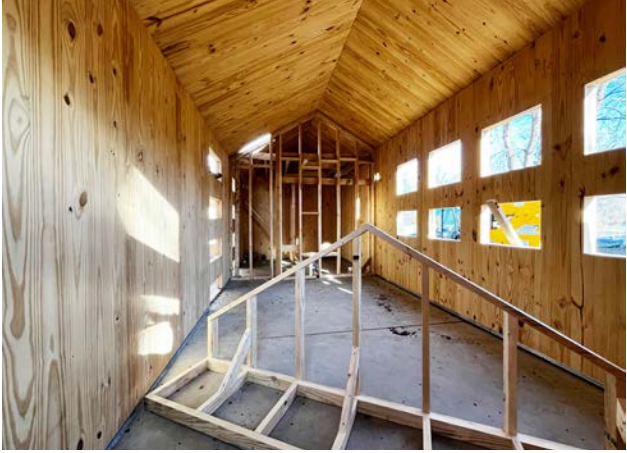
the cross laminated timber shell is complete
