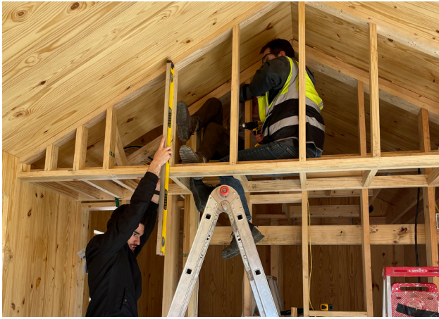
partitions, soffits, electrical, and plumbing are installed
