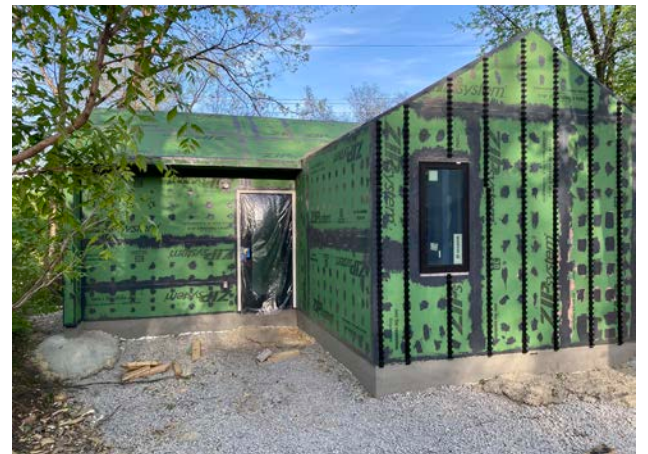
building envelop is fully waterproofed and air sealed
