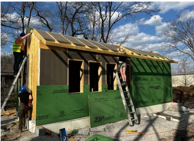
installing ZIP sheathing and continuing to install insulation
