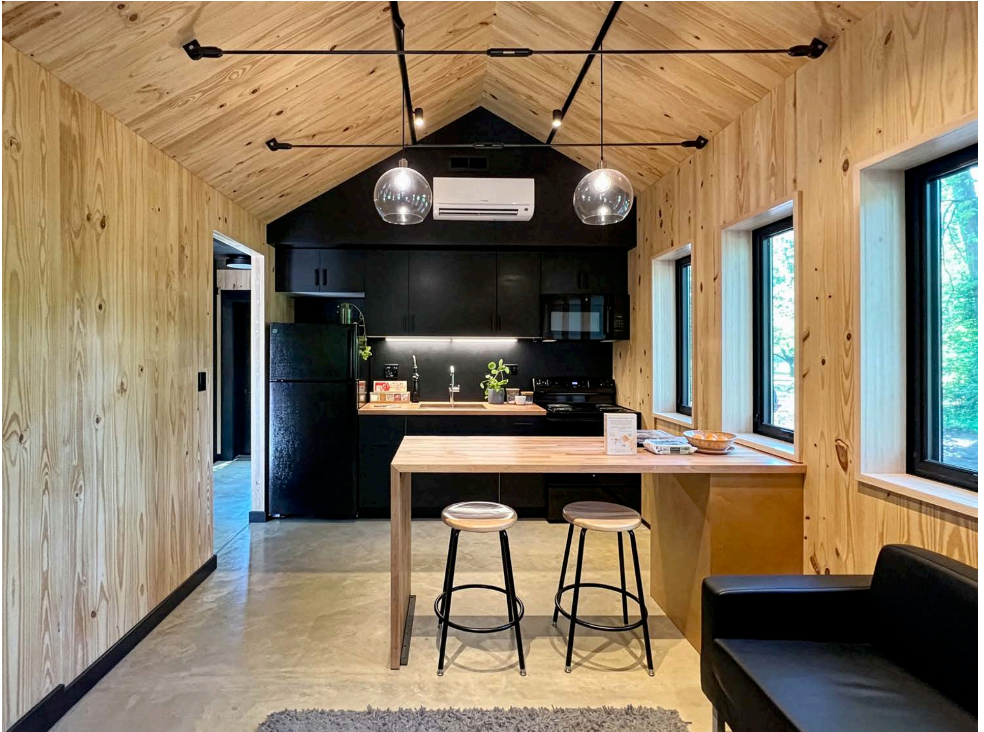
Interior view of the dining and kitchen area, seen from the living room, with the exposed cross laminated timber shell and exposed radiant-heated concrete floor
