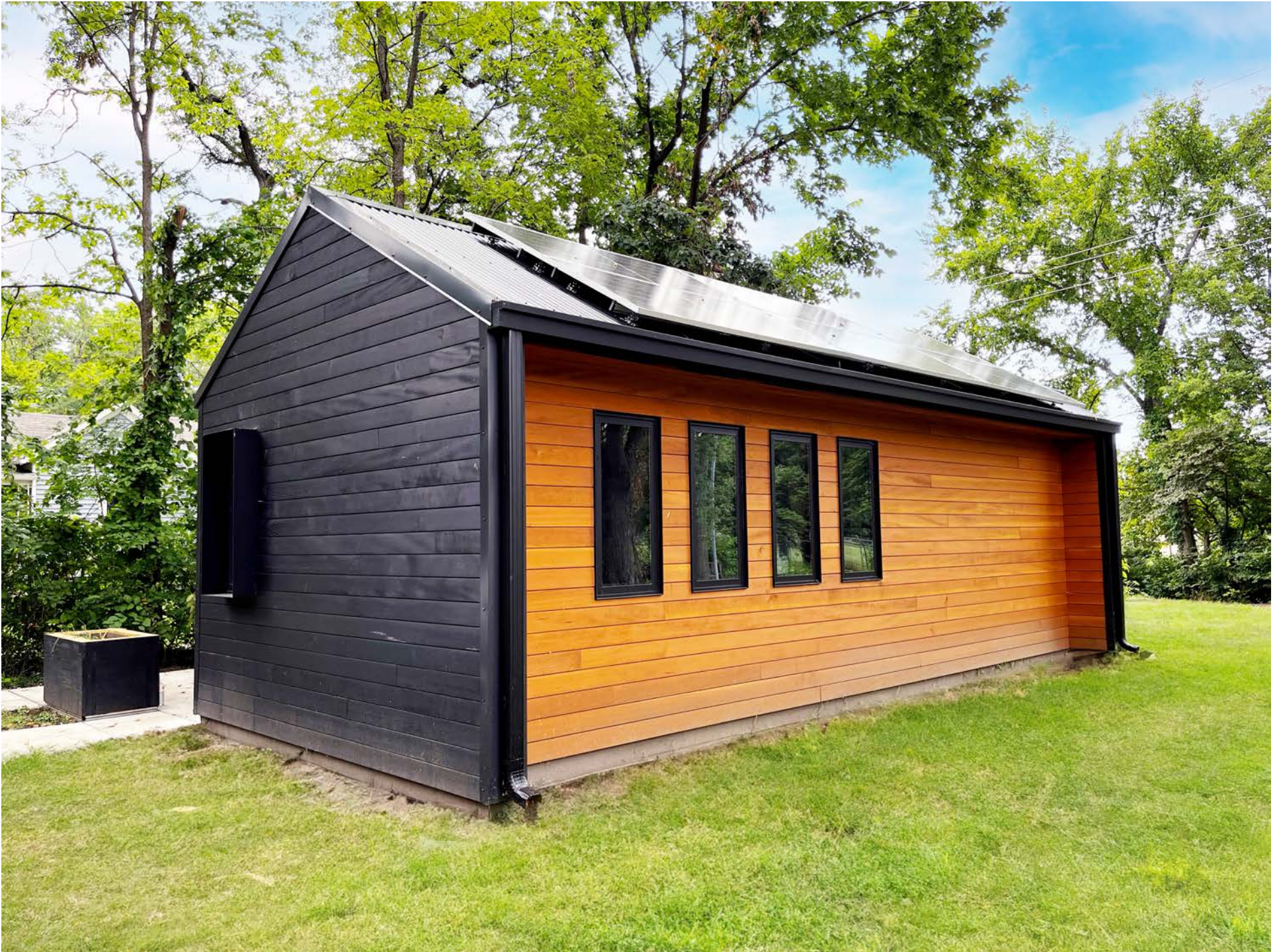
Exterior view of the southwest corner, with the large south-facing facade characterized by a warm brown wood rainscreen inset and roof-top solar panels
