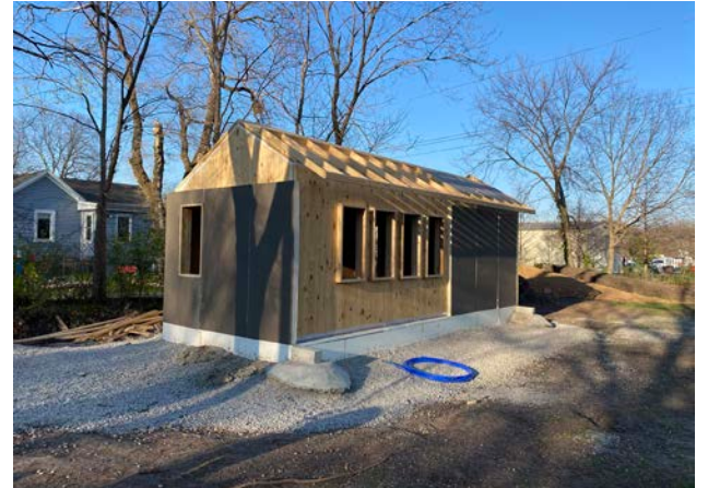
installing roof eaves, window bucks, and exterior insulation
