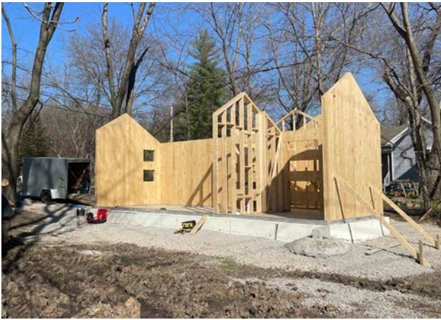
pre-fabricated interior partitions are installed as well
