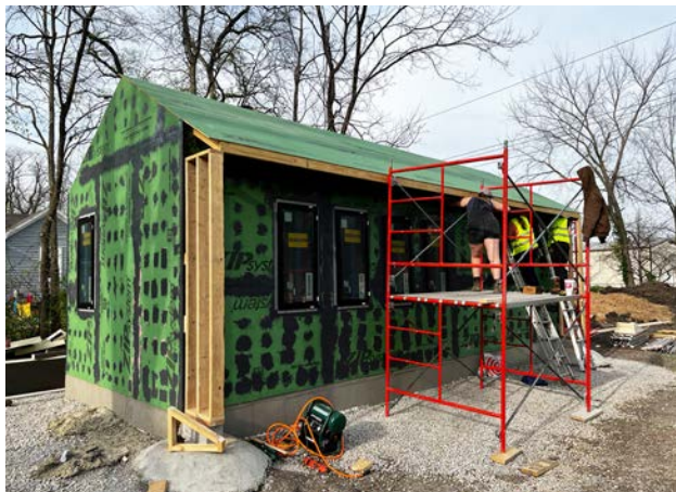
installing windows and enclosing wing walls and eaves
