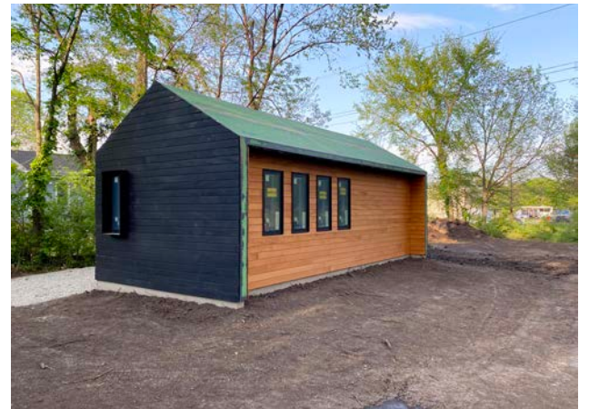
rain screen almost completed, regrading the site
