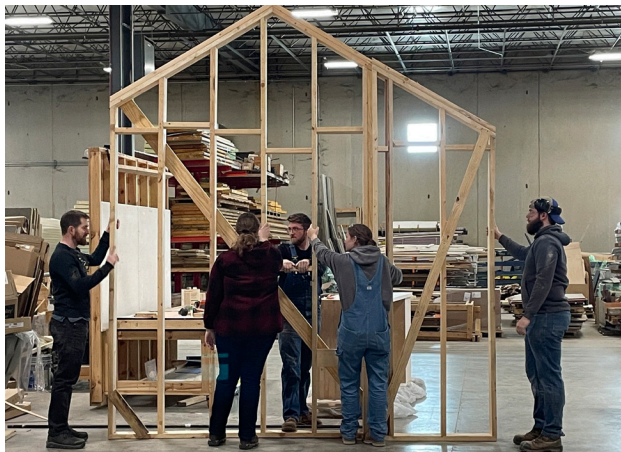
mocking up interior partition walls
