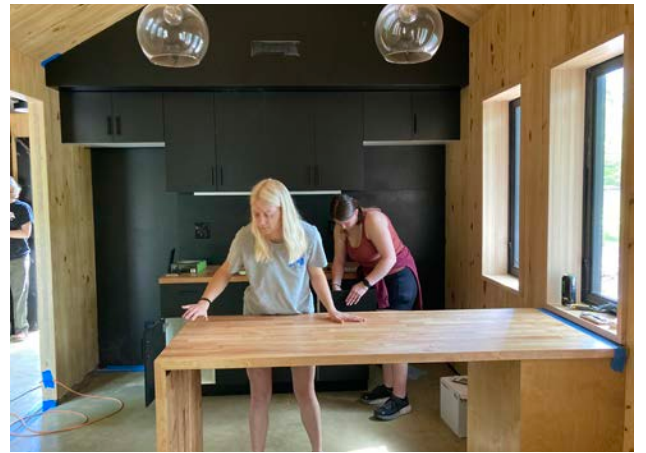
punchlist and prepping for appliance/equipment installation
