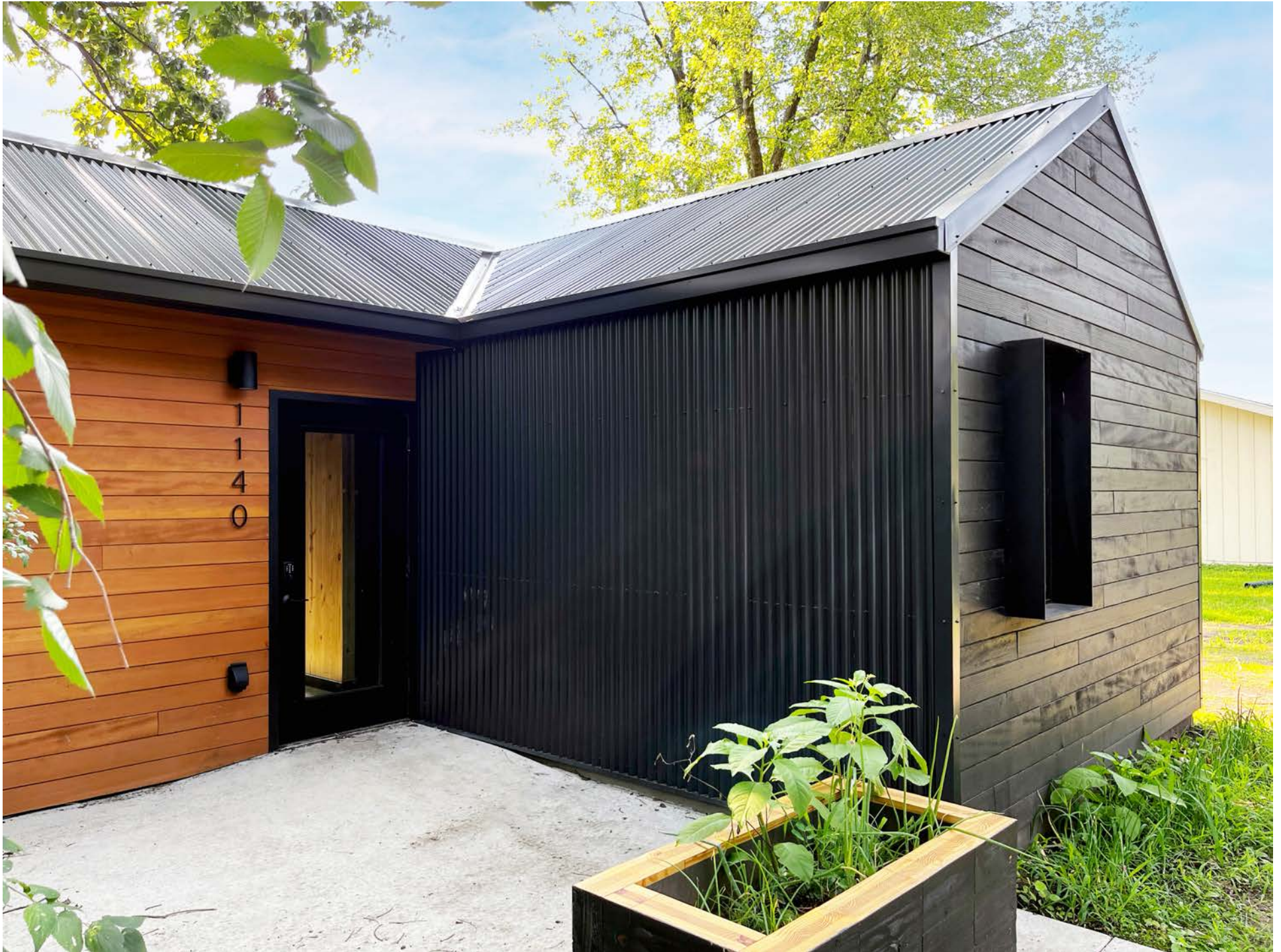
Exterior view of the entry, with black wood rainscreen and black corrugated metal panel siding on the main volume and a warm brown wood rainscreen on the inset entry wall; a CLT planter in the foreground
