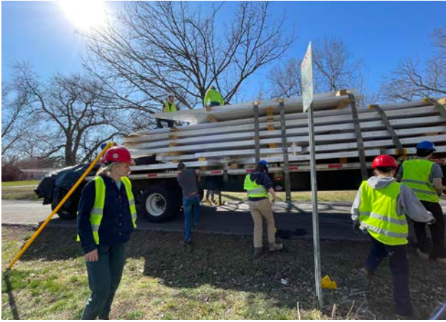
eleven cross laminated timber panels arrive
