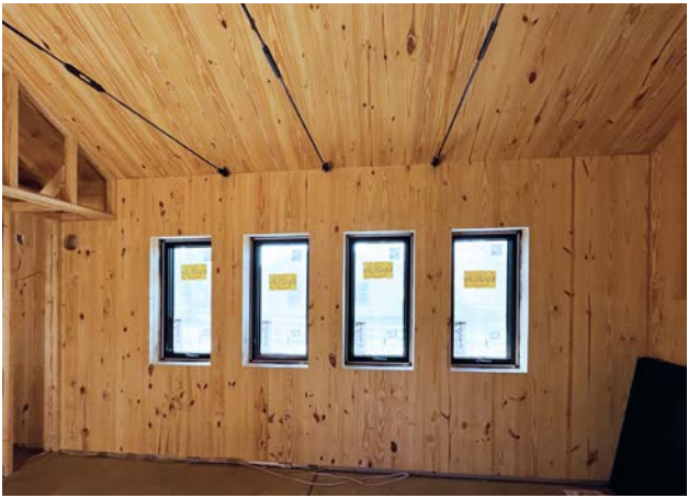
all windows installed, steel tie rods installed
