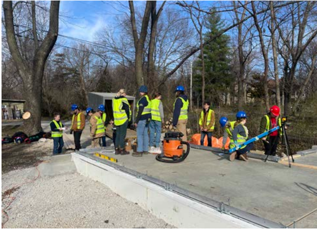
an aluminum base system is installed and leveled
