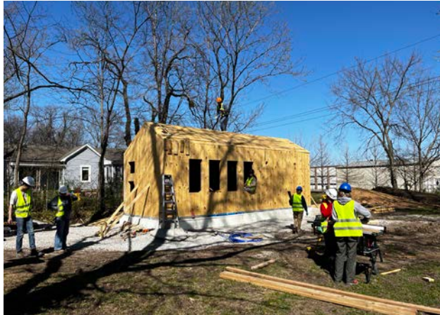
finalizing rough openings in cross laminated timber
