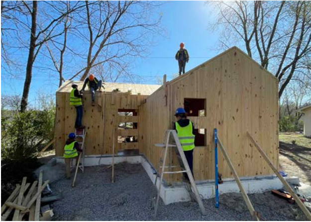
finishing attaching the cross laminated timber roof panels
