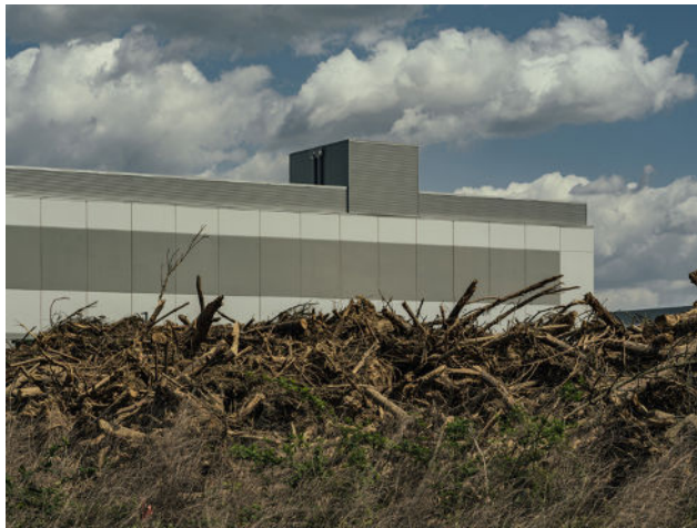
A series of photographs by Stephen Voss illustrate the disruptive and destructive nature of data center development in Northern Virginia along the Washington and Old Dominion Trail
