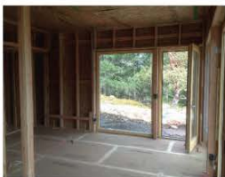
8.11.6 Open stud cavity inside the air barrier sheathing. ARTISANS GROUP
