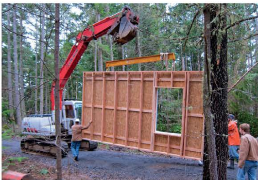
8.11.5 Placing the panelized double stud walls. ARTISANS GROUP
